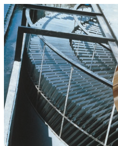
Tilted plates with hooks for water supply systems, sedimentation separators (ET, EQ)
