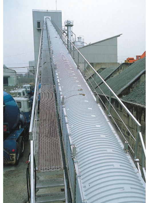
Conveyor line covers (EVX)
