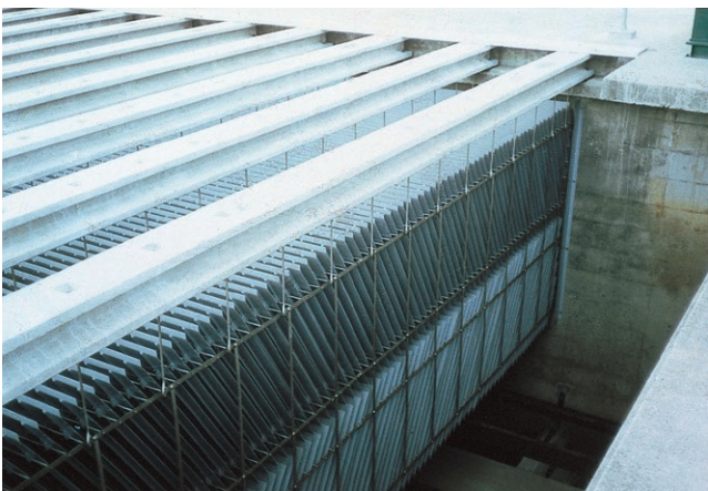
Tilted plates with hooks for water supply systems, sedimentation separators (ET, EQ)
