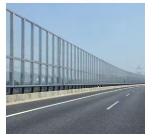
Transparent polycarbonate plates for road construction (SHIN-TOMEI EXPWY)
