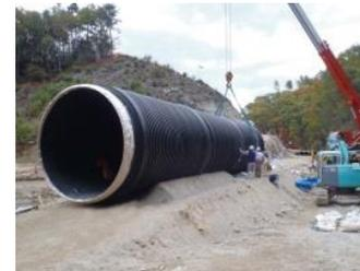
High-pressure polyethylene pipe
