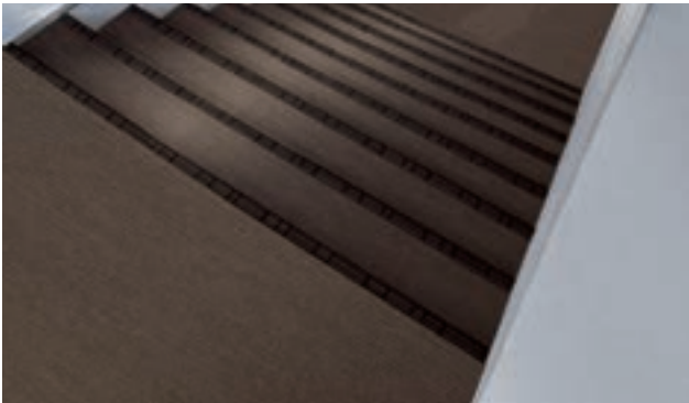
Top stair nosing: C8-837 Stair tread: 8W-837, Landing sheet: NA-837
