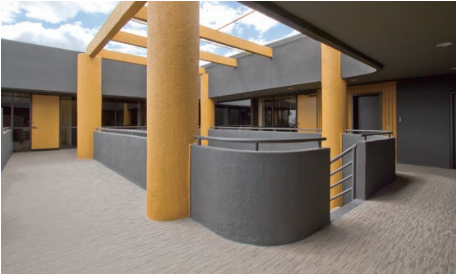
Arizona Medical Center, US (PRE82)
