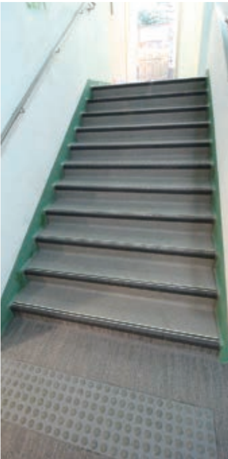
South Island School, Hong Kong (PRE81, 5C980, 5Y880)
